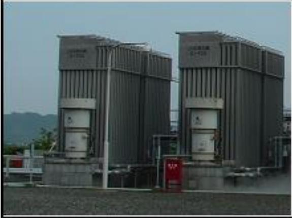
Figure 10. Ambient Air Vaporiser (Source: BV 2009)
