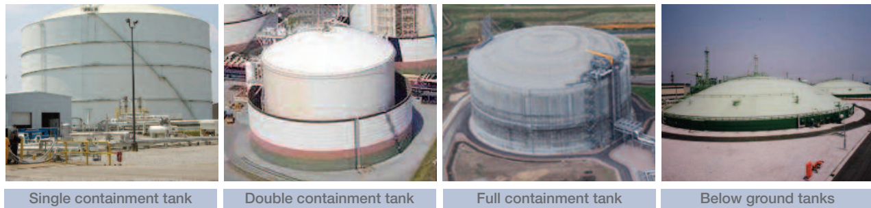
Figure 2.4 Four types of commercial LNG storage tank
