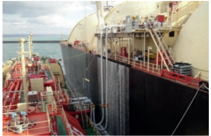
Figure 3. Flexible Hoses (Source: JAPEX)
