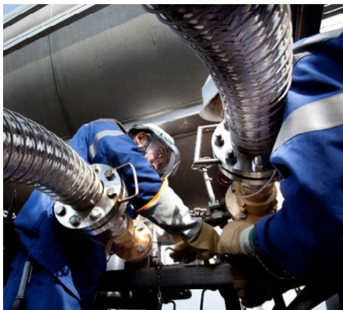
Truck loading at Montoir-de-Bretagne LNG terminal (Credit: Elengy/Cyrille Dupont)
